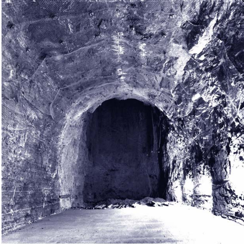
FIGURE 2-8 TUNNEL EXCAVATED IN LIMESTONE IN SOUTHERN ONTARIO
